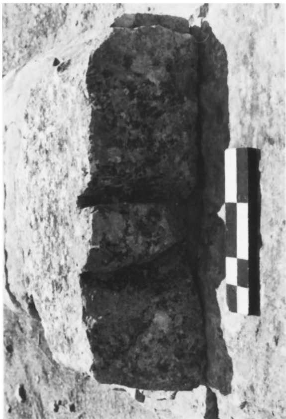
(b) 'U'-shaped lifting hole in column drum.
